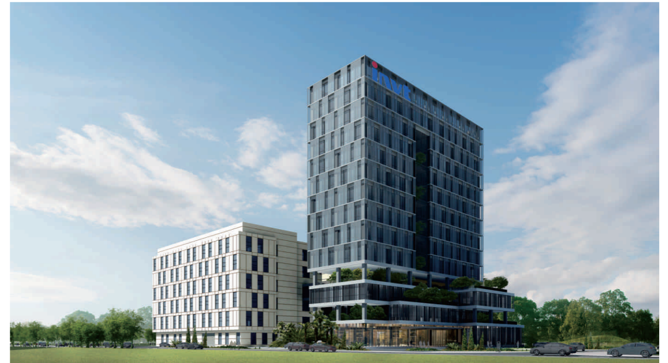
Shenzhen Industrial park
